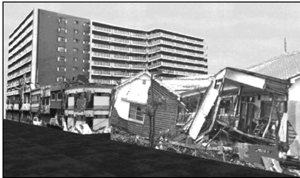
Fig. 8. Kobe City after the 1995 Earthquake (By Stefan Lisowski)
